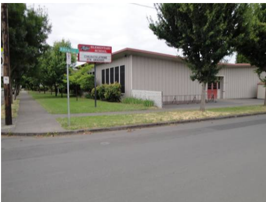
South and east elevations
