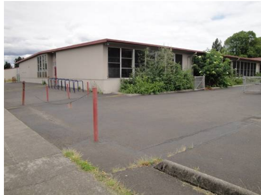
West and north elevations
