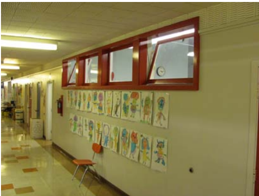
Windows between classroom and corridor
