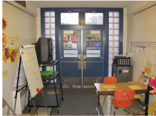
Side entry door with glass block side lights
